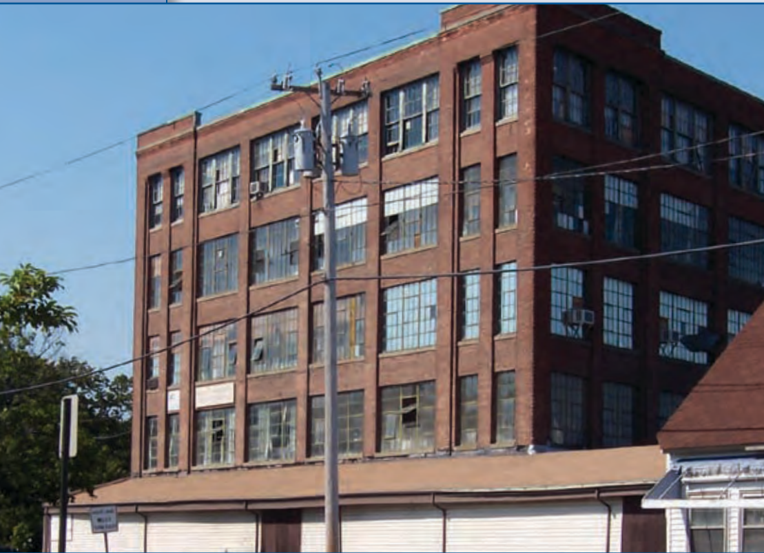
Final planning approval for the redevelopment of the historic Rumford Chemical Works property was granted in 2007.
