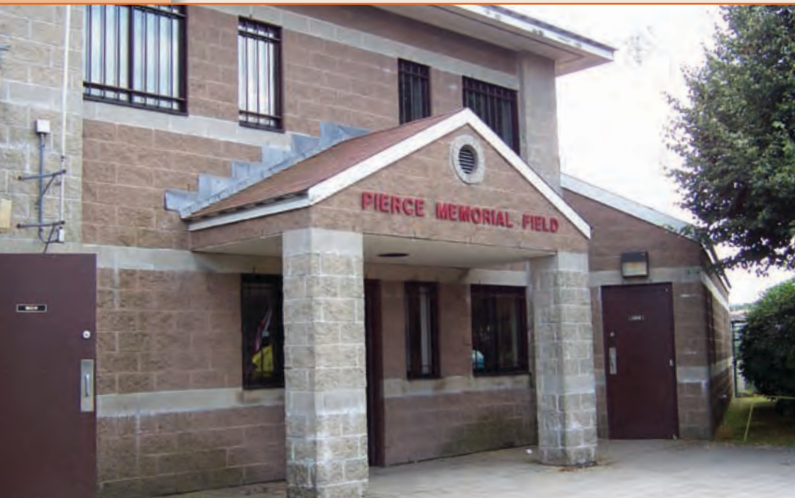
The Pierce Field Complex located in Riverside spans 26 acres and includes a fieldhouse with press box, rest rooms, storage, and office areas as well as a 1/4-mile track and stadium, baseball field, little league fields, softball field, tennis and basketball courts.
