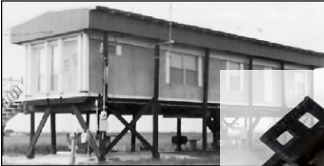
Manufactured Home Showing Cross Bracing and Foundation.
